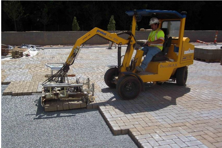
Figure 4-3. Example of Machine Installation of PICP
