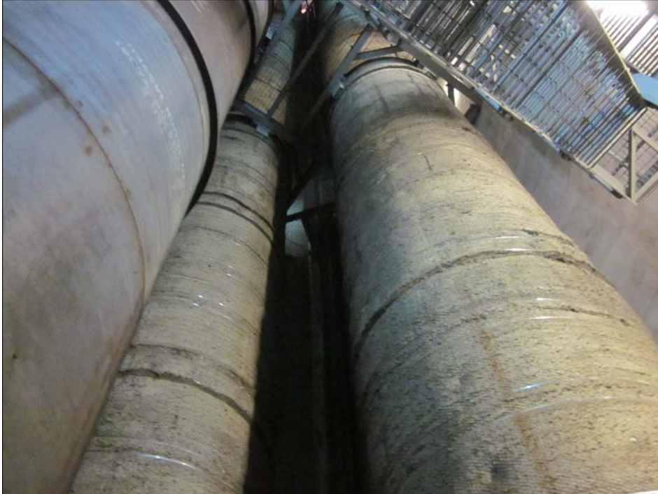
11 - outside of the 3 flues. On the left, without insulation, the Unit 3 flue.
