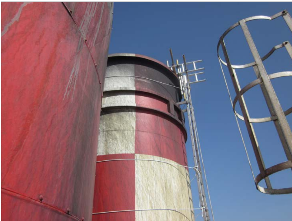
13 - red-white warning stripes on the outside of the flue Unit 3 flue still present
