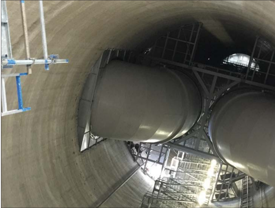
Photo 9: elbow of unit #1 on the left, no discoloration of external paint
