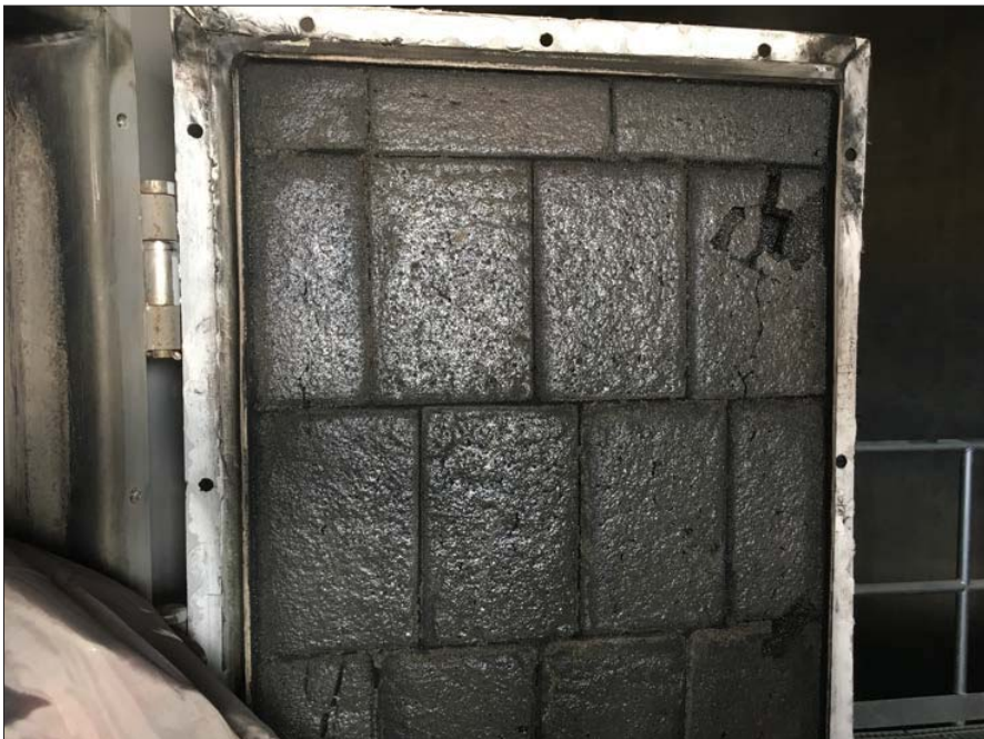
Photo 4: inspection door at landing 3 E.L. 127,2 m
