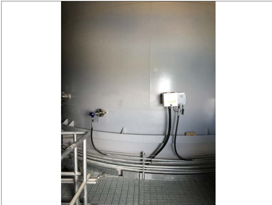
Photo 14: exterior steel liner unit #1 at CEMS level
