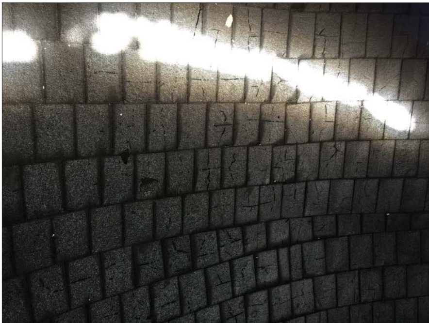
Photo 6: molten and cracked Blocks in the elbow
