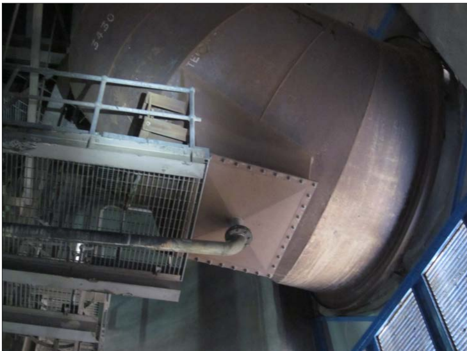
12 - view bottom flue / bend with drainage
