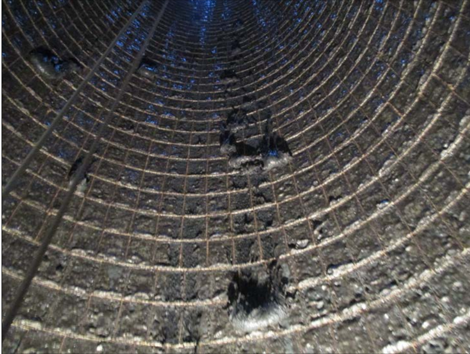
09 - view upwards halfway up the flue, with molten Pennguard Blocks
