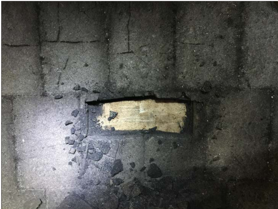
Photo 8: close up spot check target wall
