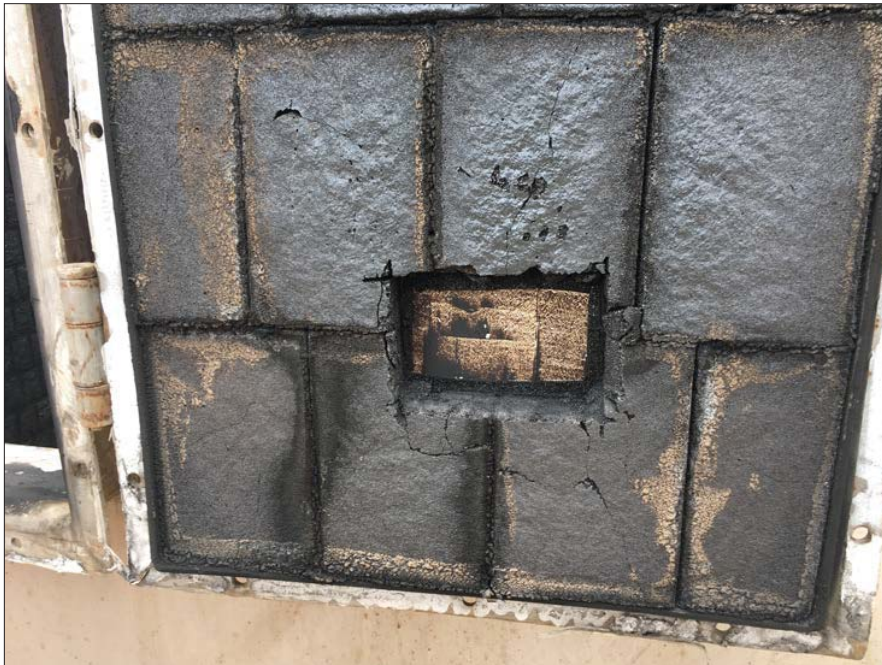
Photos 10: destructive testing of lining at inspection door of chimney flue
