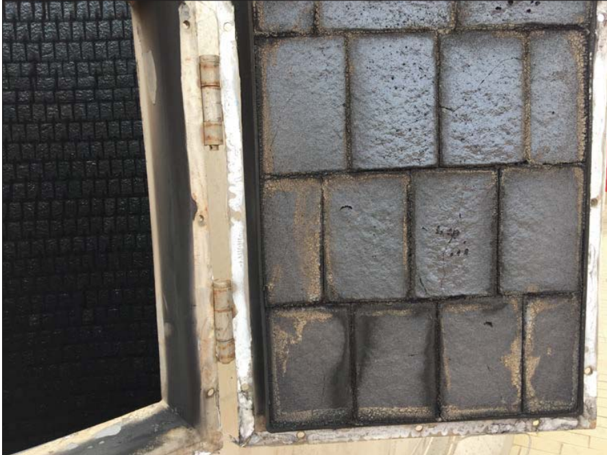
Photo 3: inspection door at the top of the chimney
