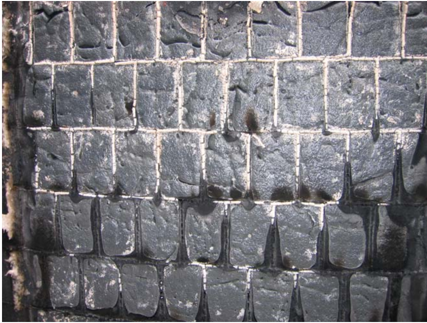
Figure 5. Pennguard wall after the ASTM E-119 test
