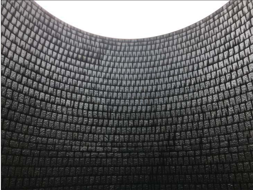
Photo 11: general overview of molten PBLs at top section
