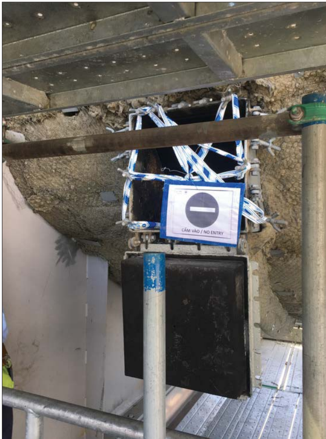
Photo 2: inspection door at chimney inlet duct E.L.42 m
