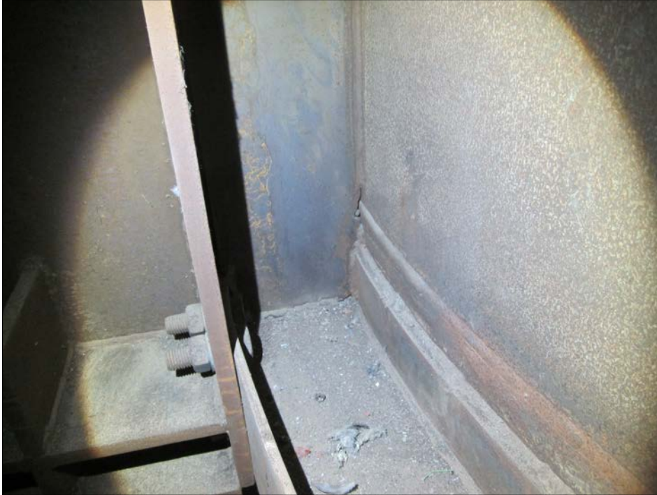
13 - close-up of a support of the flue
