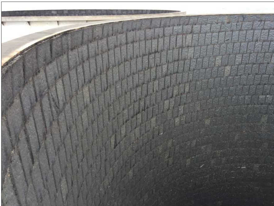
Photo 12: top Stopbar unit #1 (front), top section unit #2 (back)
