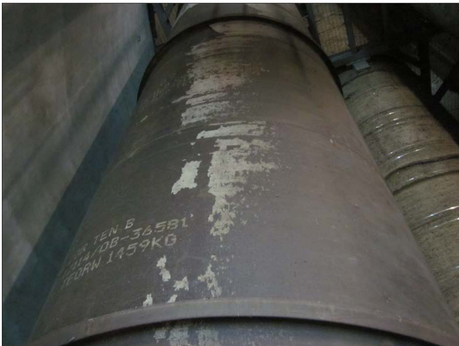
14 - outside of flue 3, half way up
