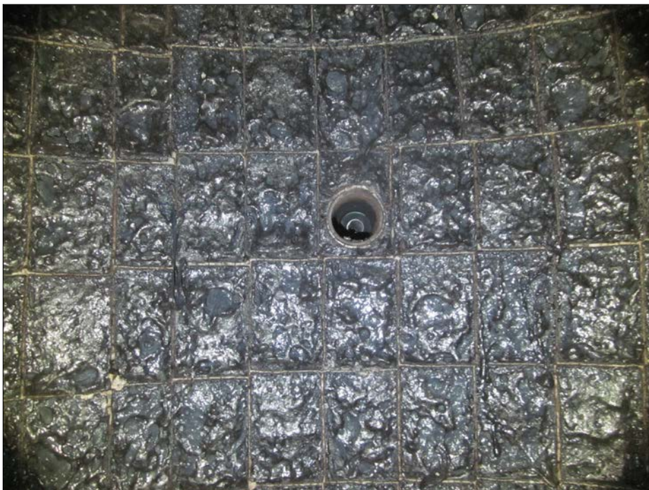
06 - Pennguard lining at level of sample ports
