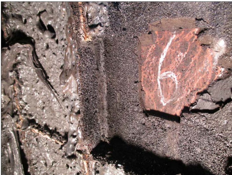
08 - spot check at +60 meters with intact back joint Membrane and Primer
