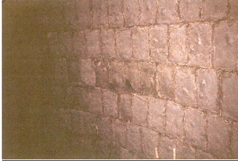
Figure 1. Surface damage to the Pennguard lining after the 1996 Endicott station fire. The photo was taken inside the chimney at an elevation of 140 feet.
