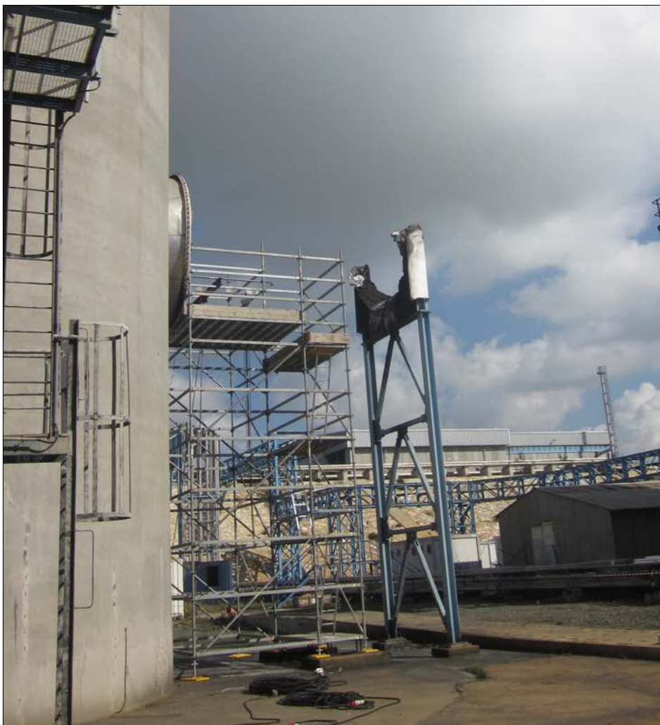
03 - scaffolding to access front of the bend
