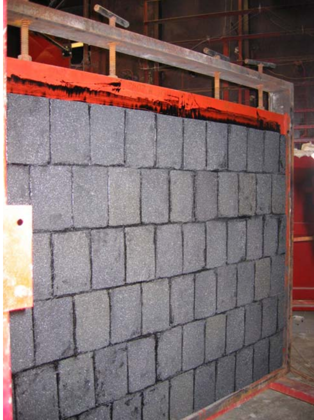
Figure 3. Pennguard lining wall before the ASTM E-119 test
