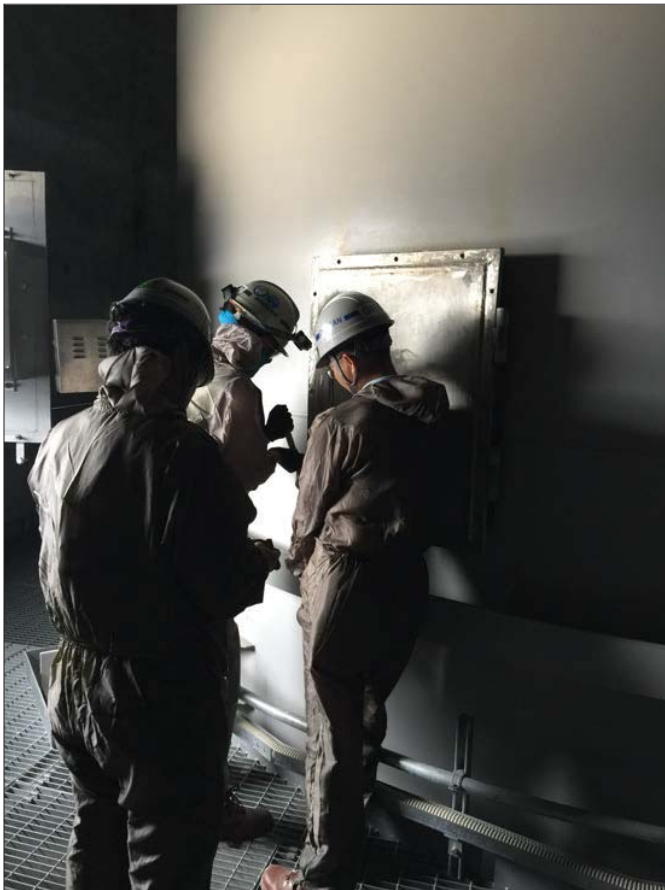
Photo 16: Doosan engineers are opening inspection door for inspection
