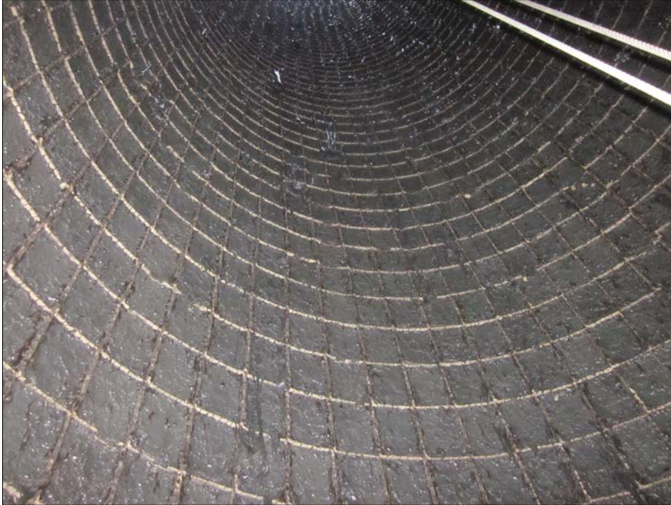
05 - upwards view taken from lower part of the flue
