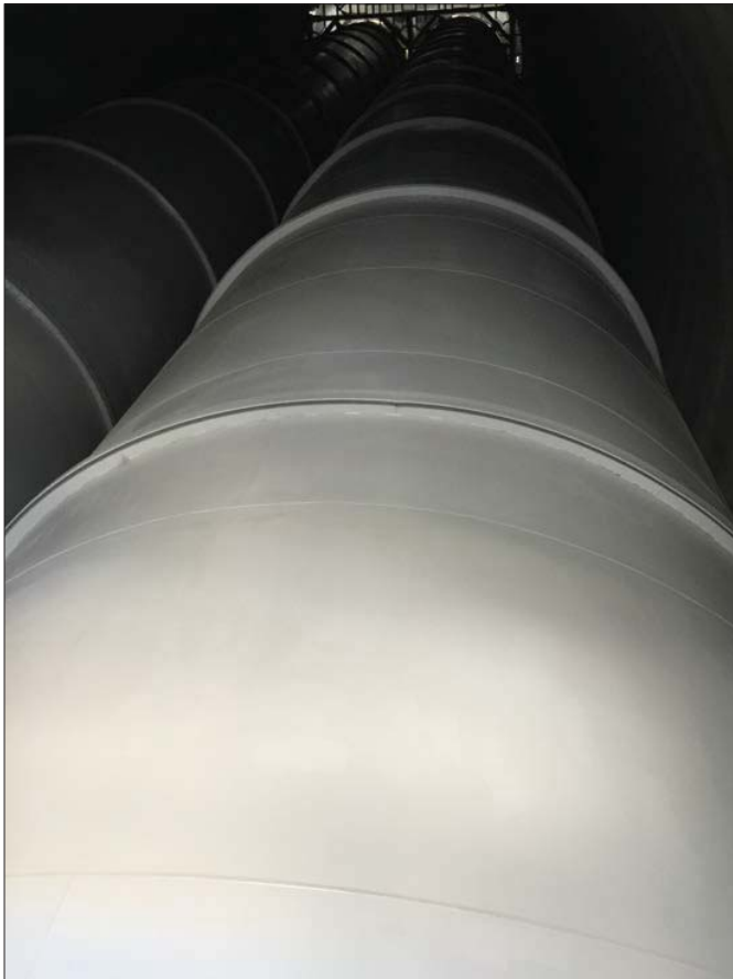
Photo 15: external paint of steel liner without damages by fire/ heat
