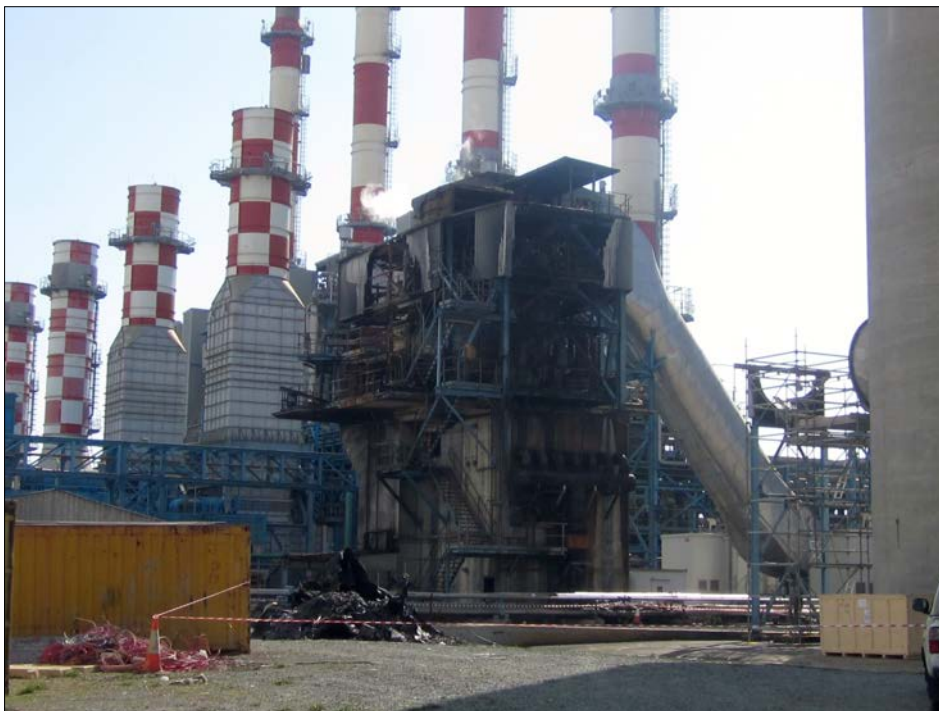
02 - heavily damaged FGD plant, FRP outlet duct completely destroyed
