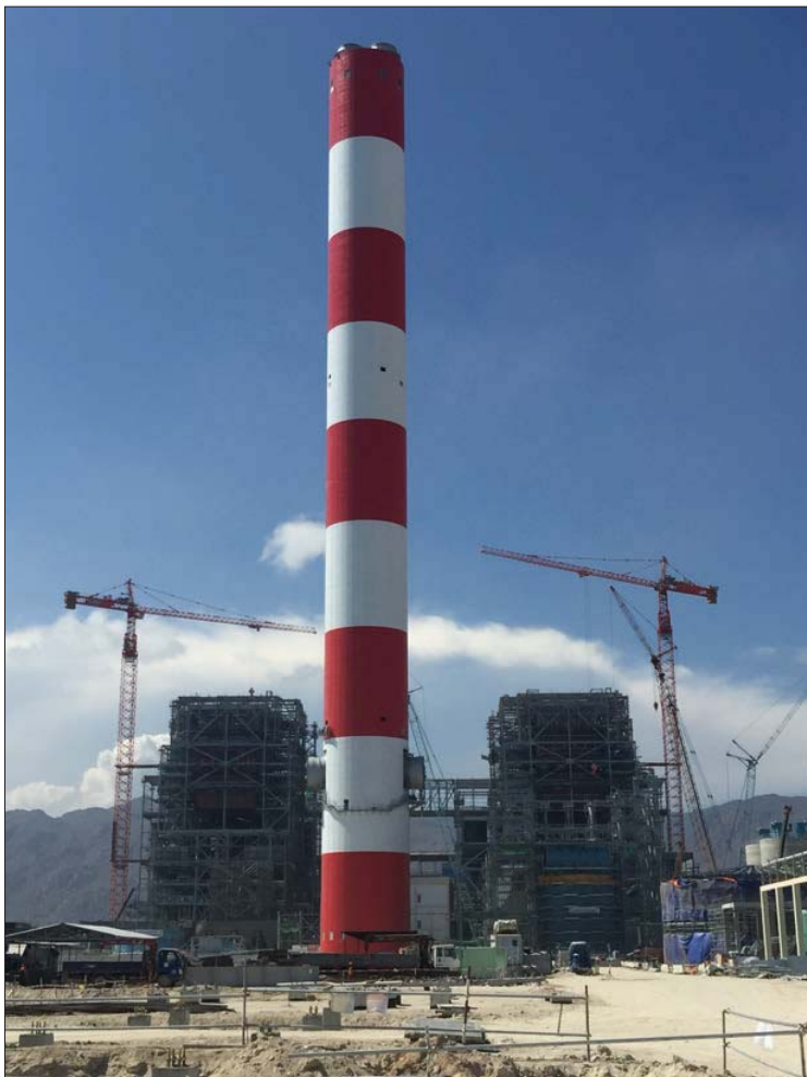
Photo 1: Vinh Tan 4 Power Station during construction phase
