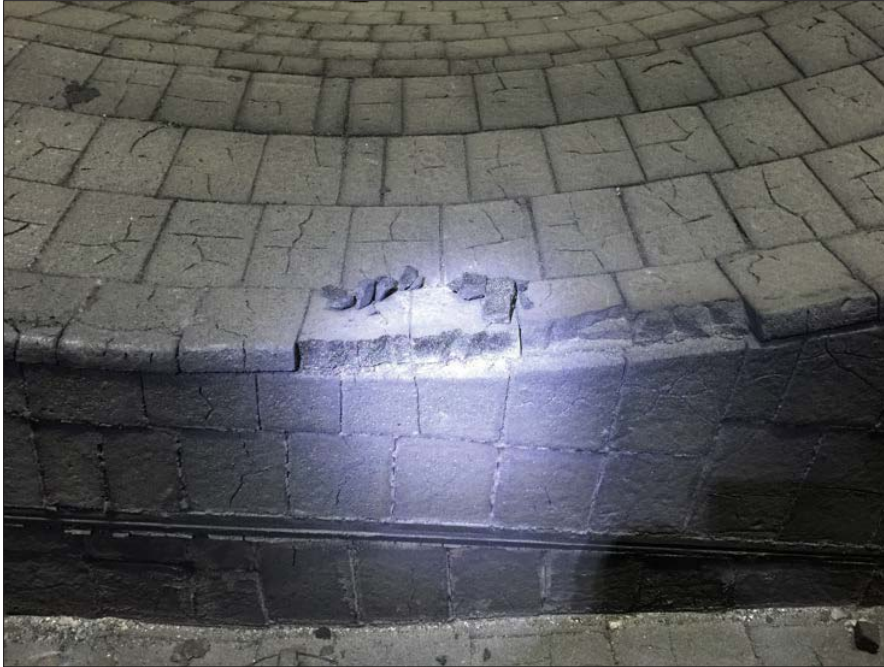
Photo 5: Pennguard lining at drainbox, loose blocks due to traffic
