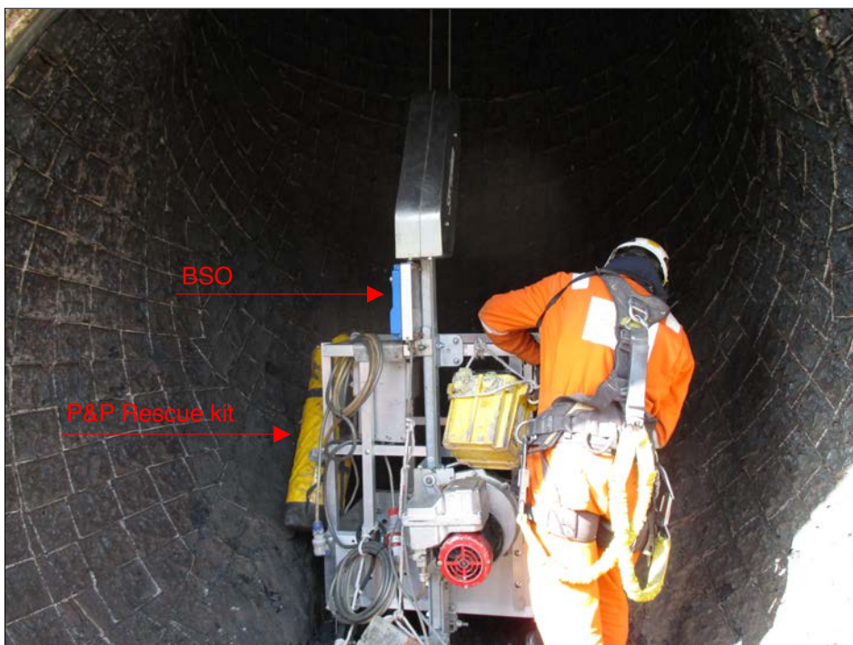
04 - 2 persons cradle suspended on a 2-rope system
