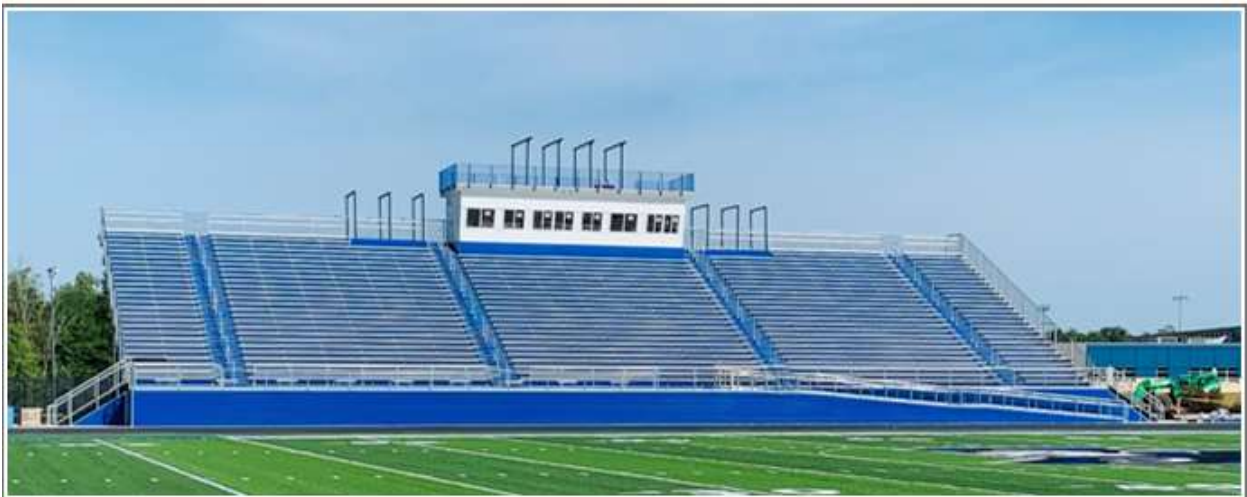
Example of ramp access to center of raised bleachers.
