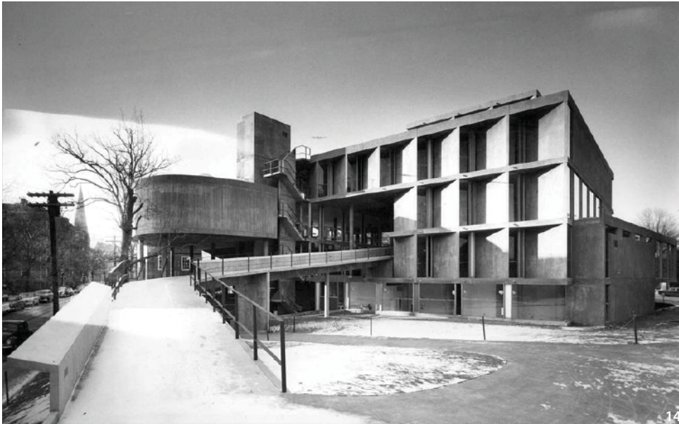
Figure 14 Carpenter Centre, Harvard University, Cambridge, Massachusetts, Le Corbusier, Architect (Source: Harvard University Archives).
