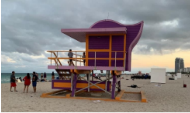
Beach lifeguard station overhang on beam
